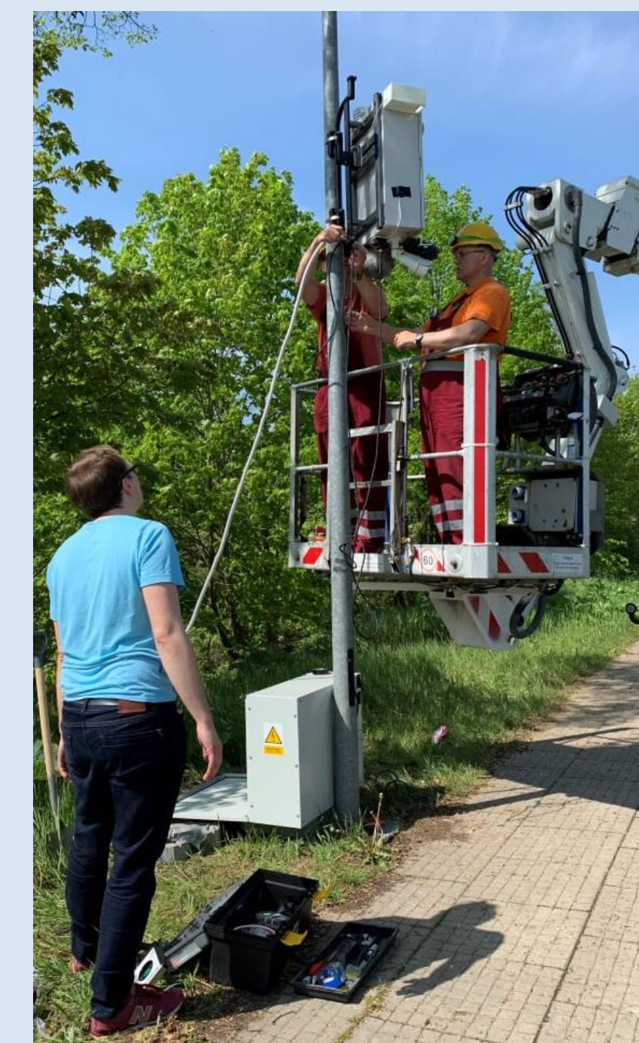
Hanging measurement module of intelligent road sign in Leżno, Poland
